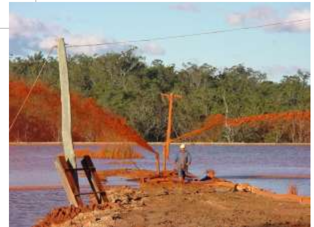
Figure 4 : Red Mud Residue being added as a Slurry to a 1500 ML Dam containing Water Polluted with High Levels of Toxic Metals
